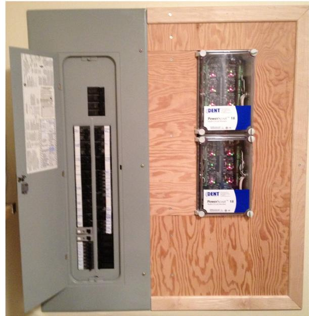
Fig. 1. Two DENT PowerScout 18 units metering 24 loads at the electrical circuit breaker panel. Measurements are read over a RS-485/Modbus communication link by data acquisition equipment (see Figure 3(a)).
